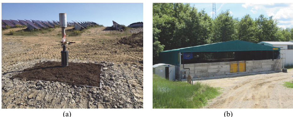
Fig. 1. Biofiltration systems: (a) biowindow, (b) biofilter
